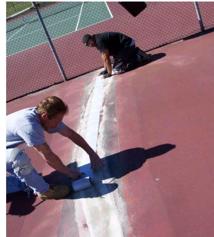
Applying RiteWay MicroSealant tape to the crack.
