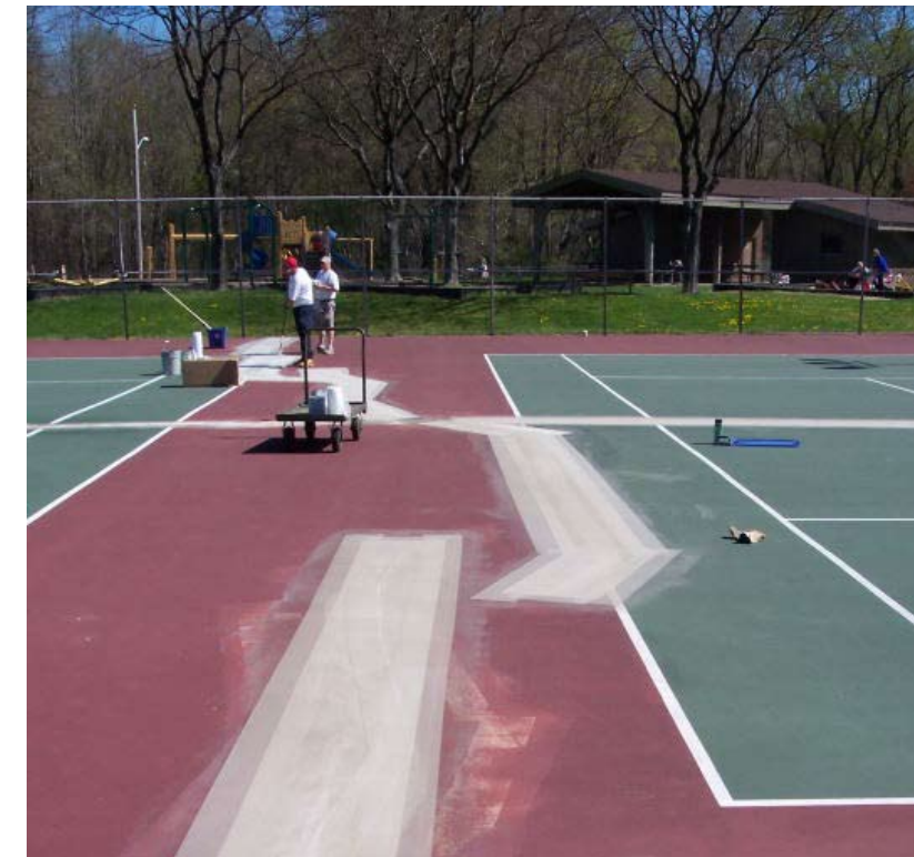
Completed RiteWay crack repair. Guaranteed for 2 years!
