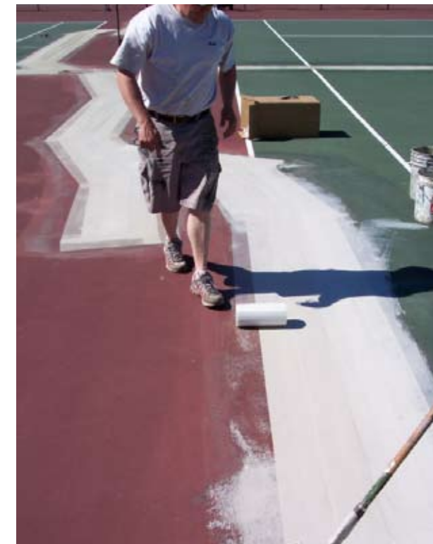
Applying bonding edge and coating with acrylic.
