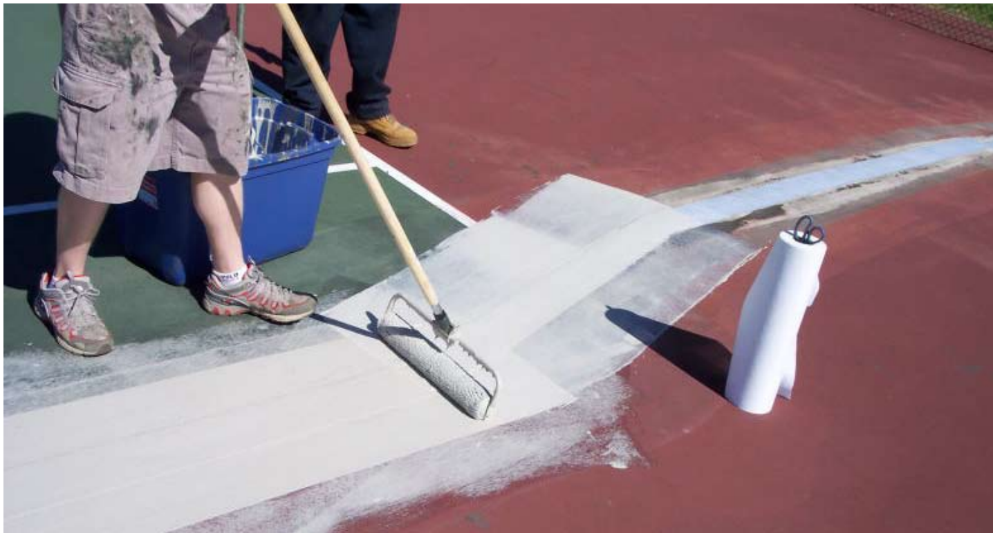
Applying acrylic to first layer of tape, then applying stress matt (fabric).
