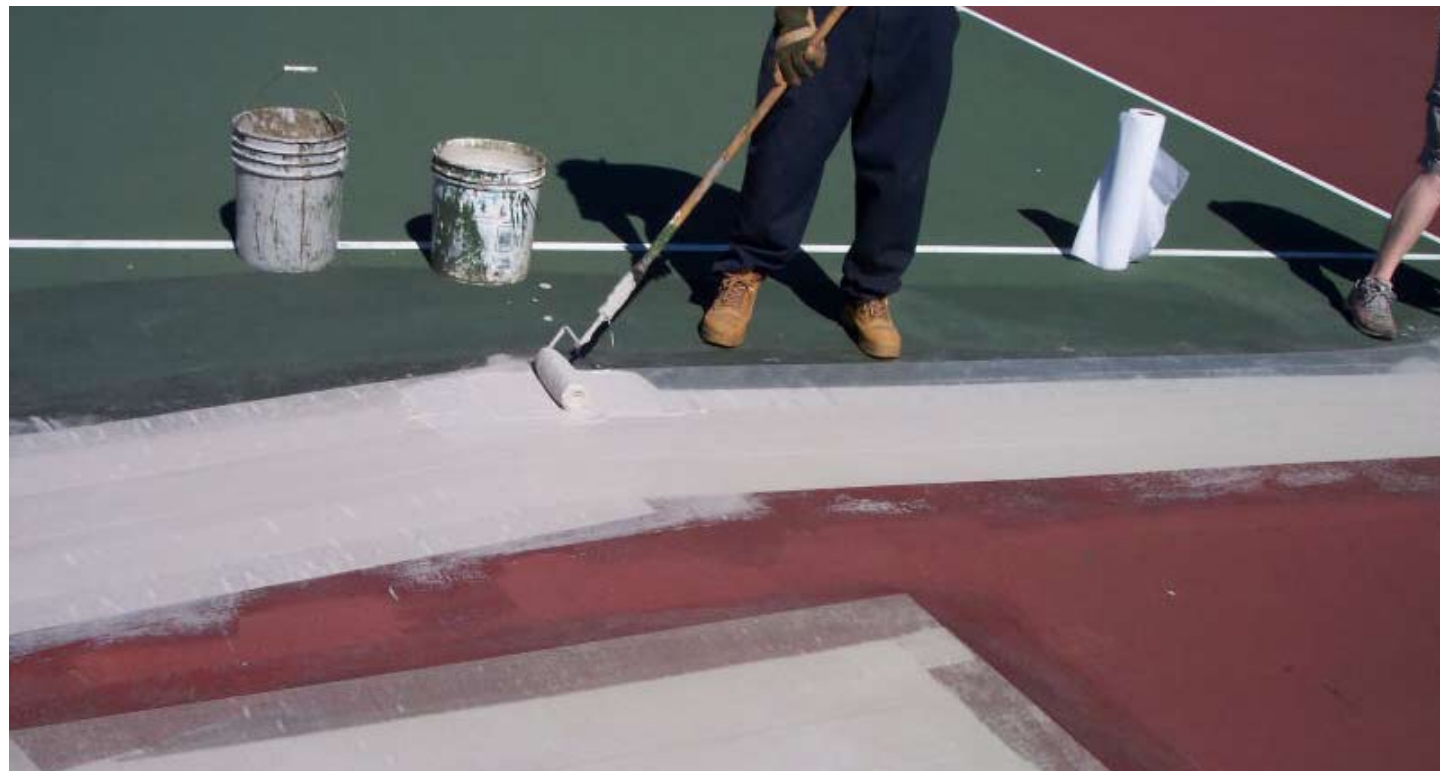
Coating the bonding edge.
