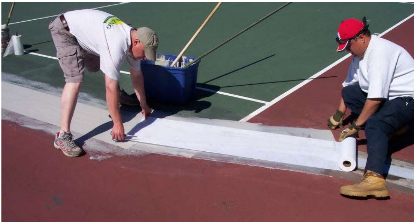
Applying stress matt with wet acrylic and no sand.
