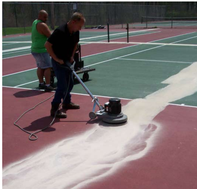
Buffing a filled crack until smooth and level.
